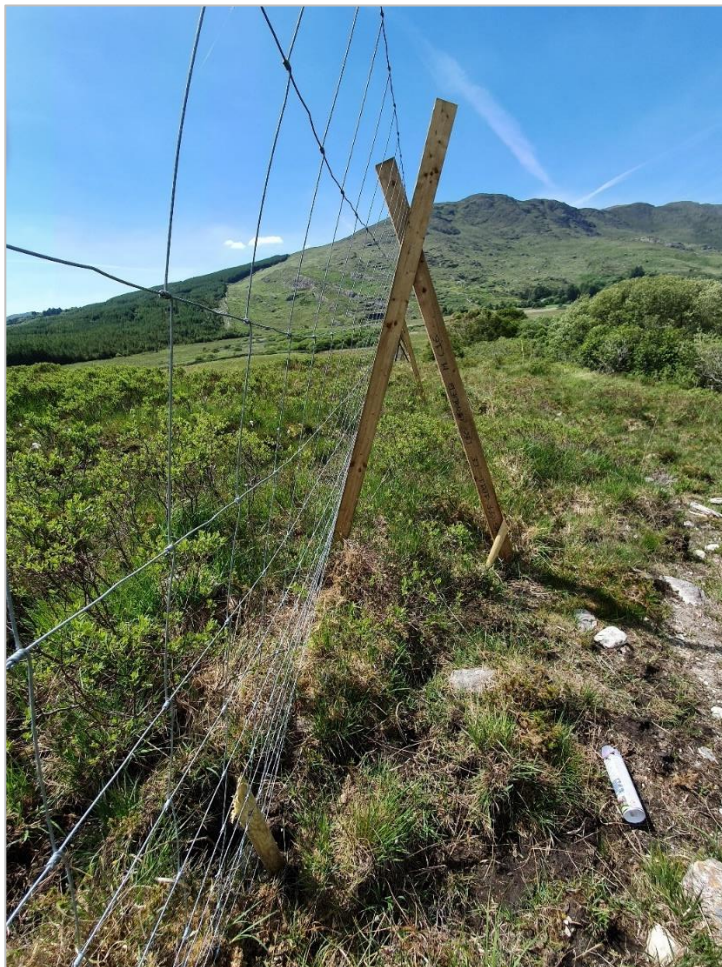
Plate 13. A-frame fencing detail showing pegging of mesh and stay to ground. Photo by Paddy Purser.
