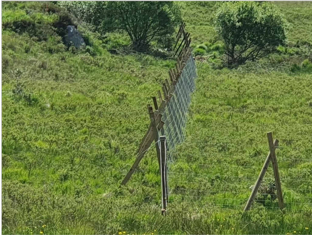
Plate 12. A-frame fencing in the Blackwater Catchment, Kenmare, Co. Kerry – note how it can “sit on top of” and “ride over” sensitive areas or difficult terrain. Photo by Paddy Purser.
